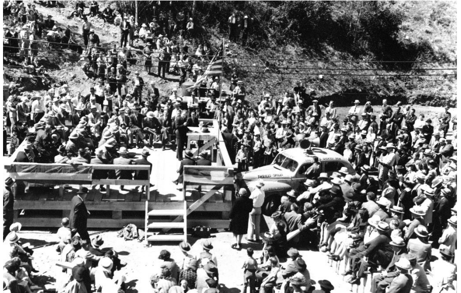
Celebration of the Adams Tunnel holing through near the East Portal in June 1940.
