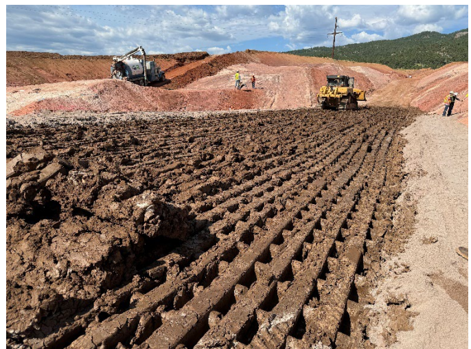
Equipment putting down clay for the Saddle Dam foundation.
