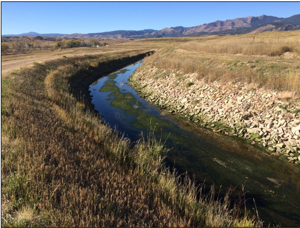
Figure 4.7. Aquatic plants in Boulder Feeder Canal prior to Fall 2015 herbicide application to dewatered canal.
