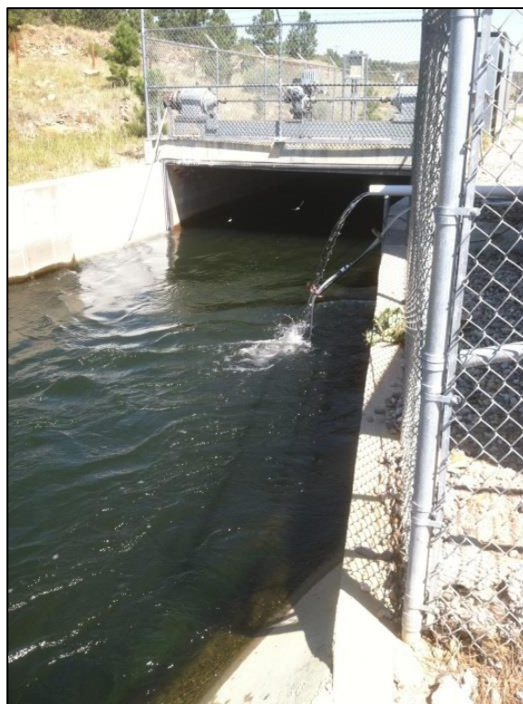
Figure 4.4 Green Clean Liquid discharge hose.
