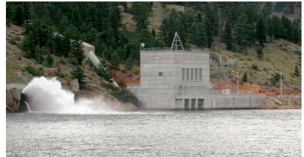
Mary's Lake Power Plant
