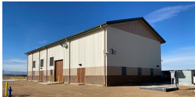
Eastern Pump Plant
