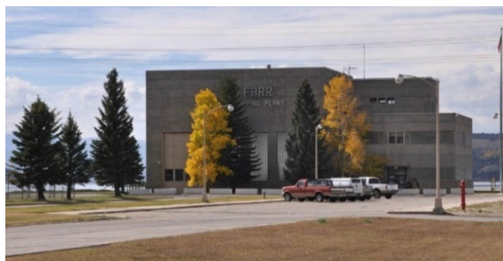
Farr Pump Plant
