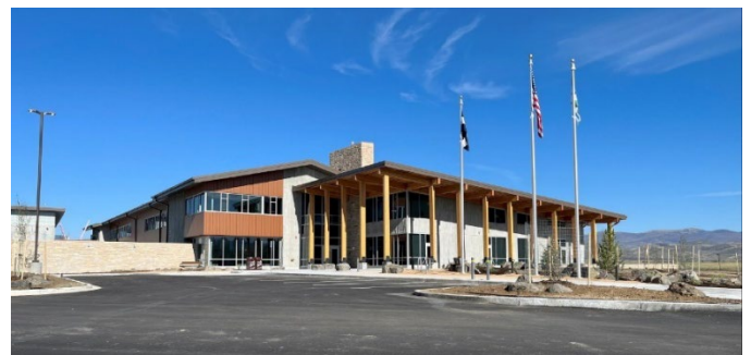
Northern Water opened its new Willow Creek Campus in Granby in September 2022. On the East Slope, Phase II construction began on a new wing for the main administration building.
