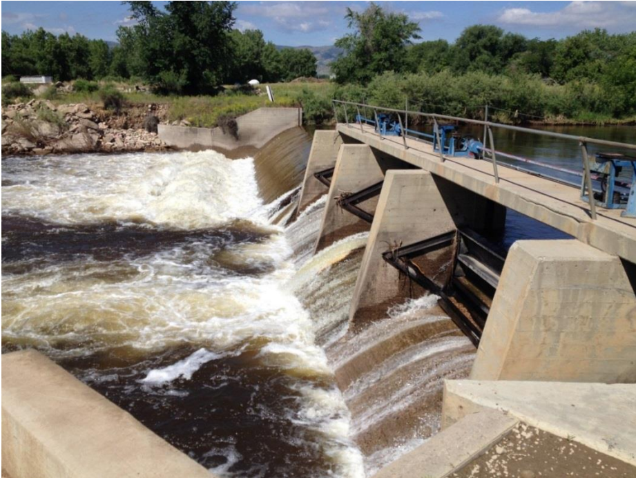
Figure 32. Existing Larimer-Weld Diversion Structure
