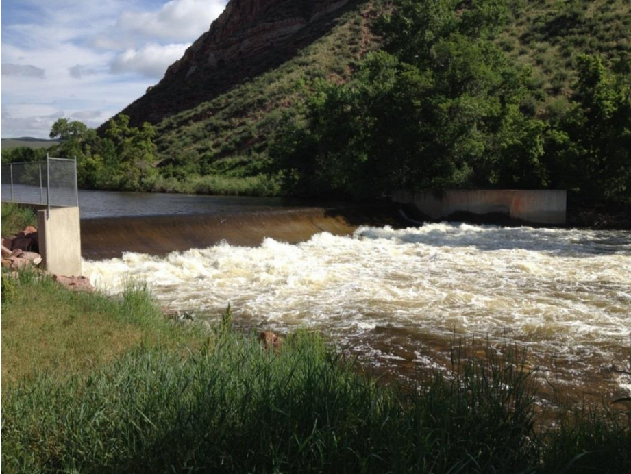
Figure 31. Existing Watson Lake Fish Hatchery Diversion
