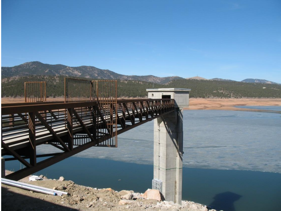
Figure 8. Multi-Level Outlet Tower at Carter Lake
