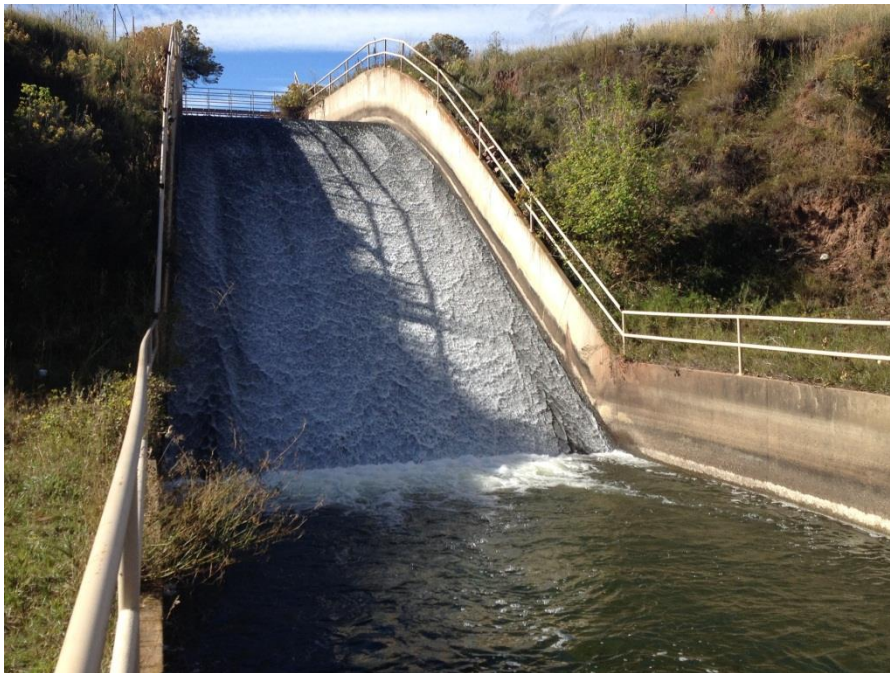
Figure 9. Hansen Supply Canal Discharge Structure to Poudre River
